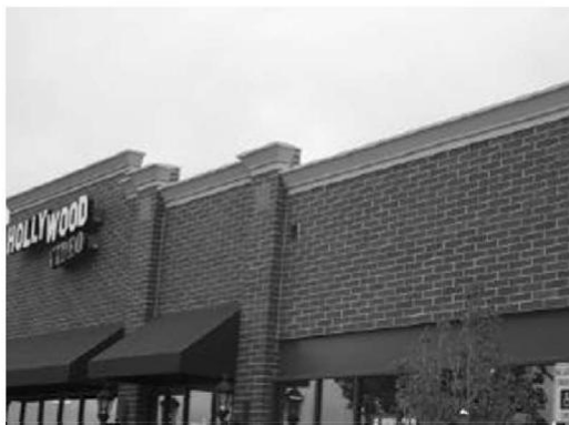
Figure 5: Parapet walls with cornice treatments are used to disguise flat roofs. The image on the right illustrates a tall, thin parapet wall that is prohibited.
