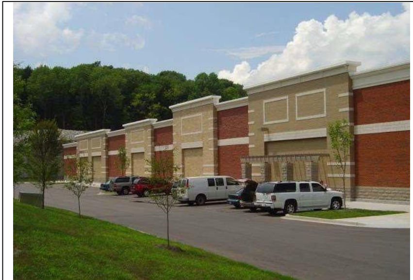
Figure 2: This figure shows two methods of using architectural features to create wall surface relief on wall elevations that are not the primary elevation.
